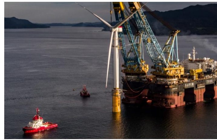
Assembly and installation of wind power
