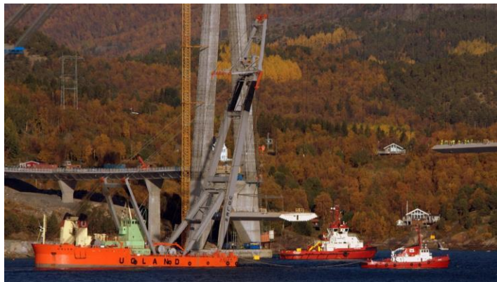
Construction work and inshore assistance
