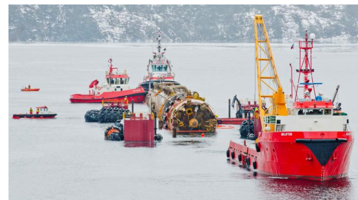
Decommissioning of offshore structures
